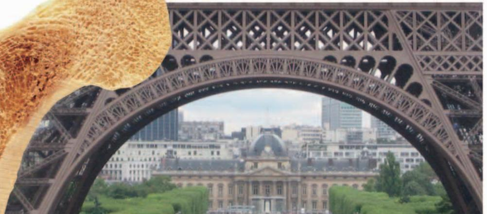
▲ EIFFEL TOWER, FRANCE The arch at the base of this tower supports its weight, helped by the criss-cross pattern of metal struts.
